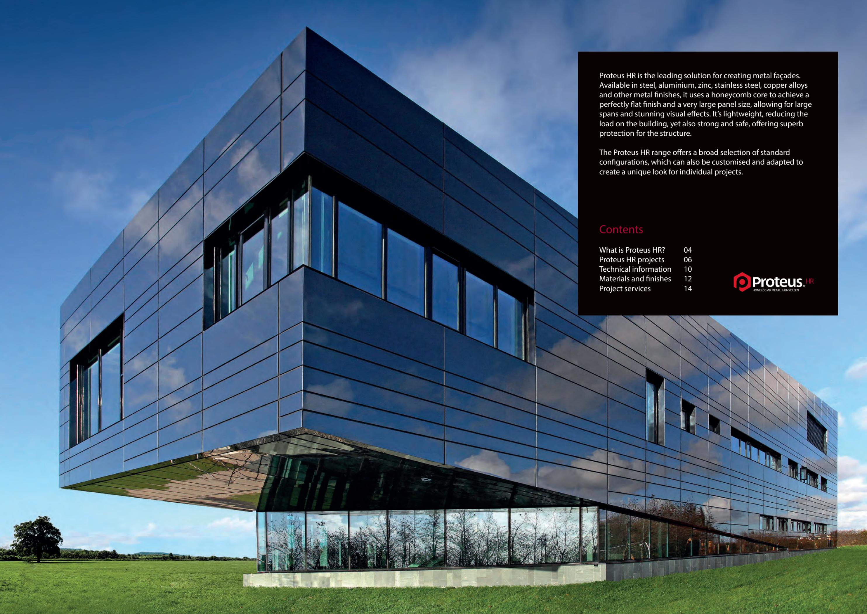
Proteus HR is the leading solution for creating metal façades. Available in steel, aluminium, zinc, stainless steel, copper alloys and other metal finishes, it uses a honeycomb core to achieve a perfectly flat finish and a very large panel size, allowing for large spans and stunning visual effects. It's lightweight, reducing the load on the building, yet also strong and safe, offering superb protection for the structure.
