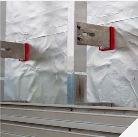
Stage 1 Helping hand brackets and vertical rails are installed at specified centres to the substrate.
