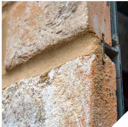
Stage 6 Set all joints to nominal 10mm, the joints should then be filled with pointing mortar and tooled to finish.
