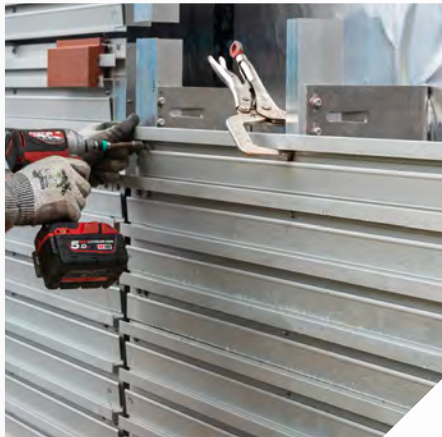
Stage 3 Stack the following carrier onto the previously fixed carrier and fix again at the specified centres.
