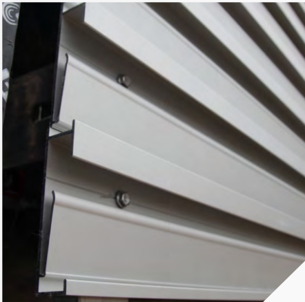
Stage 2 Position the starter carrier horizontally and ensure it is level before fixing in position.
