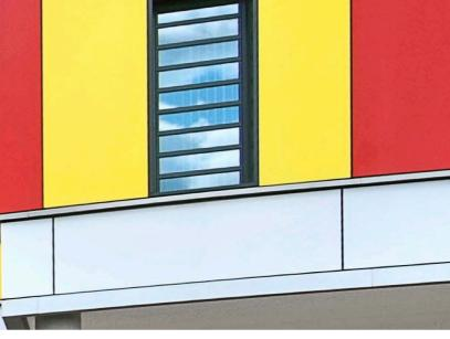
Please contact Proteus regarding requests for non-standard material widths. Panel lengths of upto 7.2m can be manufactured from coil material however please note some materials are only available in standard sheet lengths.
